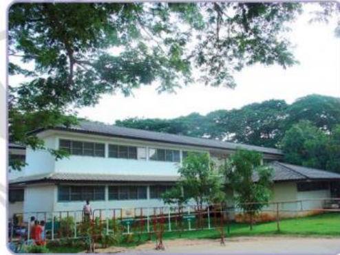
One of four buildings of the house for patients' relatives
